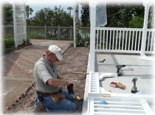
Jay Regehr, Santa Rosa County Master Gardener, supervised the construction
